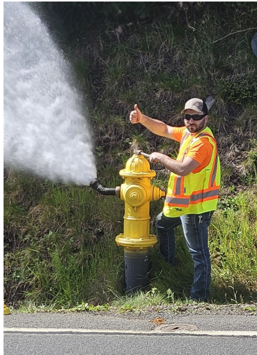
New Employee Wesley Jiroch Implements the Flushing Program
